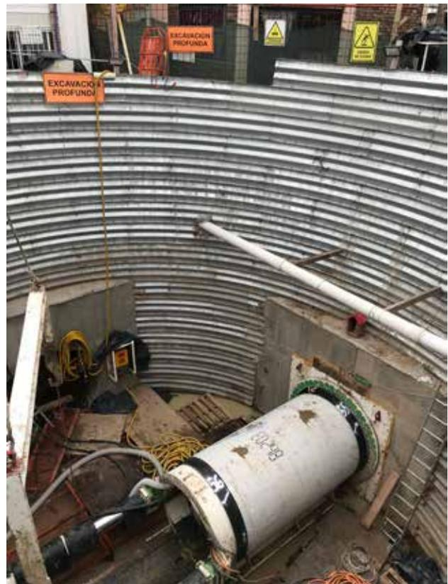
times polymers, before removal with a screw conveyor. In EPB machines the excavated ground is collected in a chamber and transported out of the tunnel mainly in wagons pulled by a winch, short trains or pumped with a thick matter pump. This micro tunnel boring machine is mainly used in cohesive soils.
