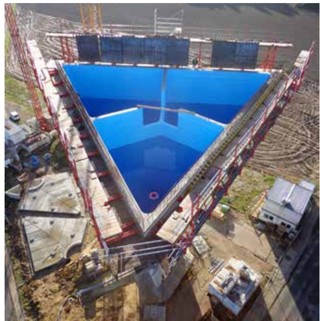
Water tower Beersel, Belgium: Sikaplan® WT-4220.
