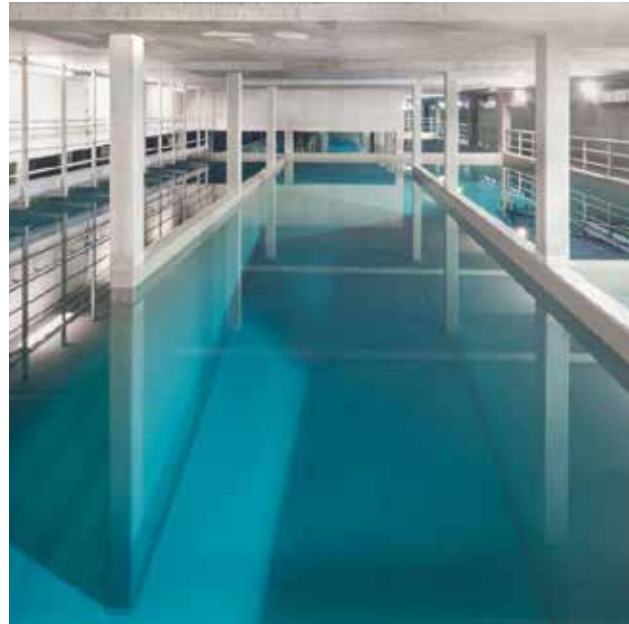
Drinking water treatment plant Kluizen, Belgium: Sikalastic® M 808
