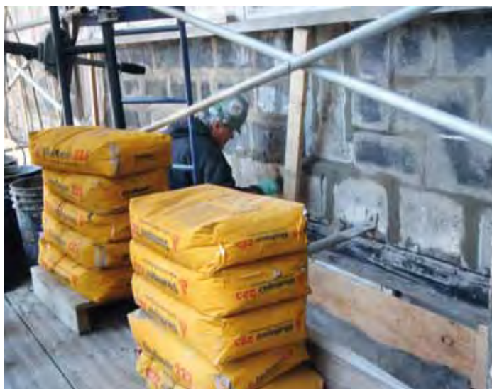
Repair mortar SikaRepair®-223 was selected to repair and patch the mortar joints, cracks and voids of the existing concrete wall structure to provide a uniform substrate before applying the membrane.
