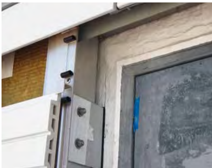
Sikagard®-560, a waterborne vapor permeable membrane was applied as a water and air barrier before installing the insulation and the new exterior rain screen cladding system.
