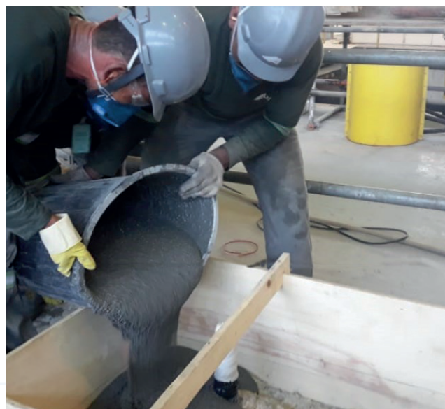
Application of epoxy grout Sikadur®-42 BR.
