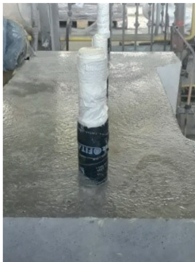
Detail of the base after execution with Sikadur®-42 BR.
