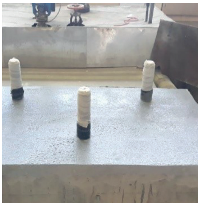
New turbine base, made with Sikadur®-42 BR.
